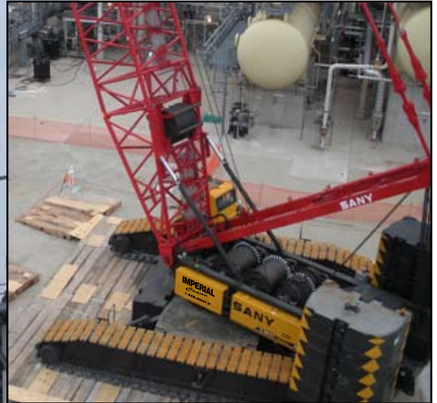
355 ton Sany setting 93,000 lb. fin fan for CITGO'S ULSD project.
