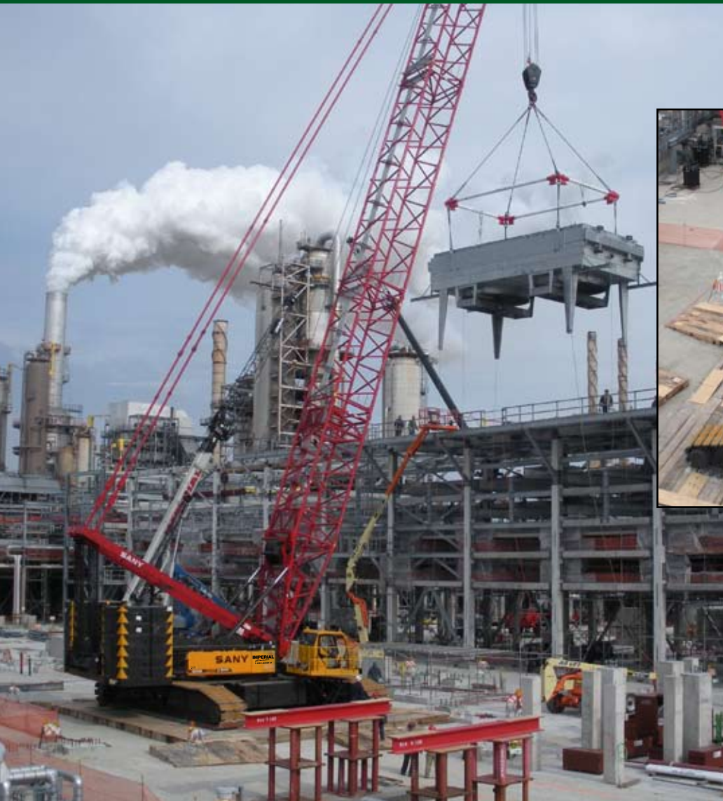
355 ton Sany setting 93,000 lb. fin fan for CITGO'S ULSD project.
